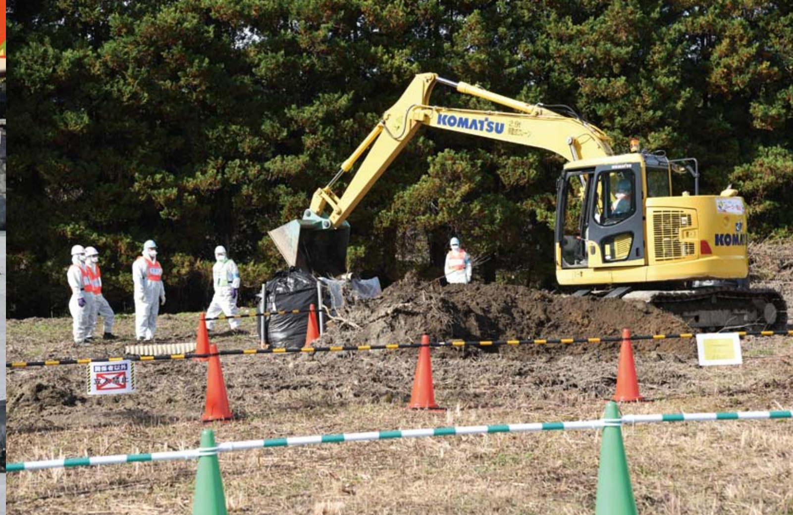
above: The Ministry of Environment organized explanatory meetings for residents about temporary disposal facility. below: Full-fledged construction begins on a temporary disposal facility in the town.
