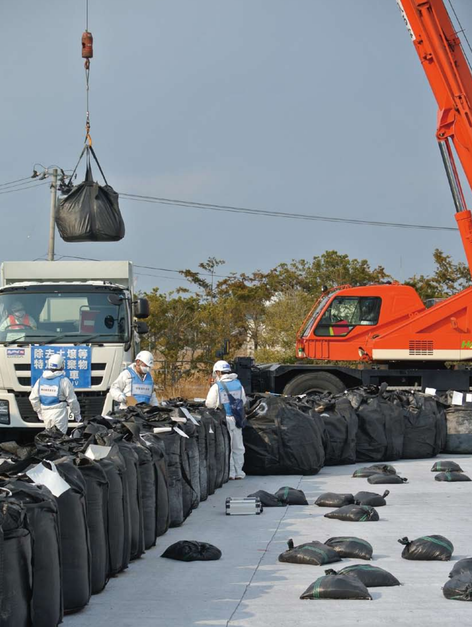
Decontamination waste is carried to a provisional storage place of a temporary disposal facility.
